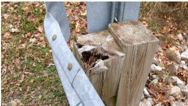
Offset Block- Deteriorated at East Barrier
