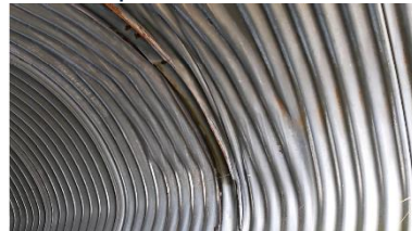
East Pipe- Dislocated Joint
