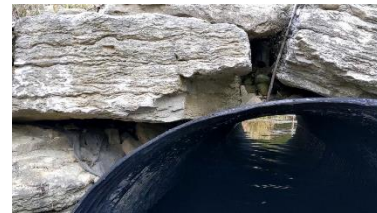
West Pipe, South end- Voids in Top Fill
