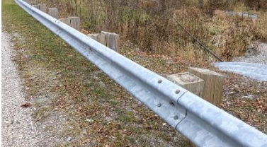
Panel laps in Wrong Direction
