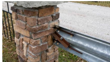
Connection of Guide Rail to End Brick Post
