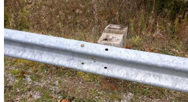
Panels missing bolts at post
