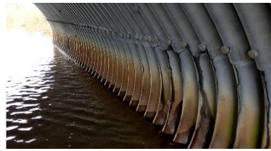
Barrel- Corrosion Line
