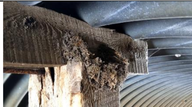
South Pipe-West Post Crushing
