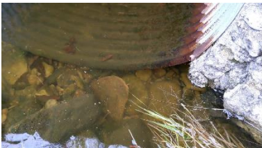
End of Barrel at East- Undermining
