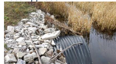
West Barrel- Sediment Build up Overtop Barrel
