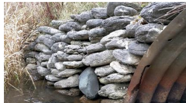
North Pipe-Retaining Wall at West
